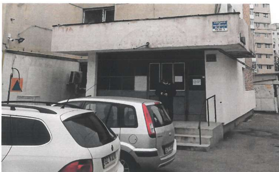
F5. Usa acces principal in bloc
