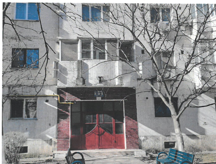
F6. Usa acces principal in bloc
