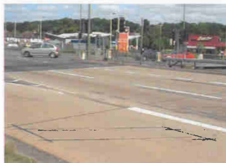
Figura 49 – Bucle inductive instalate in asfalt (exemplu)
