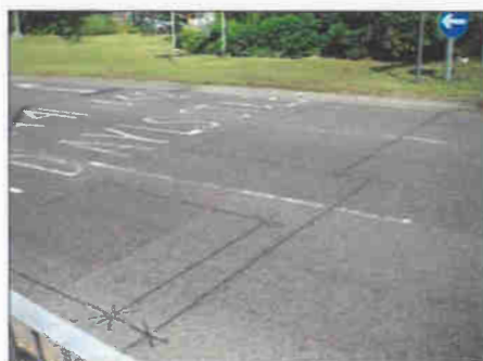
Figura 49 – Bucle inductive instalate in asfalt (exemplu)
